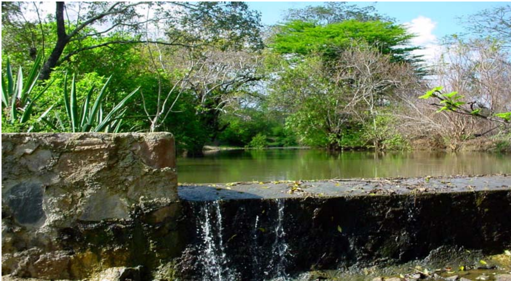
Photo 2: A sand dam in the wet season
