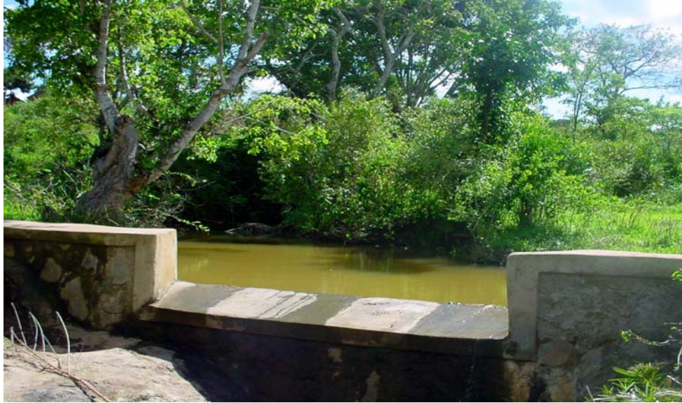
Photo 5: A sand-storage dam during the wet season
