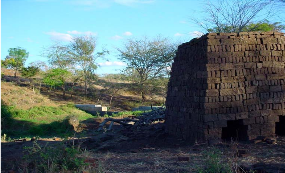
Photo 8: A sand dam and newly created bricks
