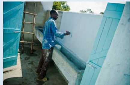
A KESSP latrine being painted Photo: CARE/Brooks Keene (2009)
