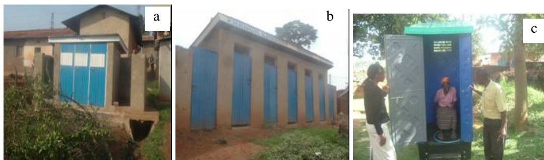
Figure 2: a and b) VIP communal latrines in Mulago III & Bwaise II parishes, c) An 80 year old woman who is a beneficiary from an Ecoo-loo Ecosan toilet installed by SSWARS in Kyebanda parish.
