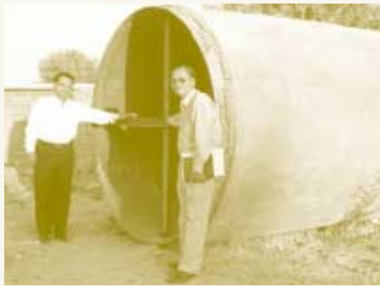
WITH FUNDS FROM THE BOND ISSUE, THE AMC CONSTRUCTED A NEW WATER PUMPHOUSE AND PIPELINES TO SERVICE 60% OF THE CITY'S POPULATION.
