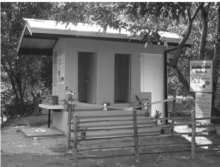
An ecosan toilet in a school
