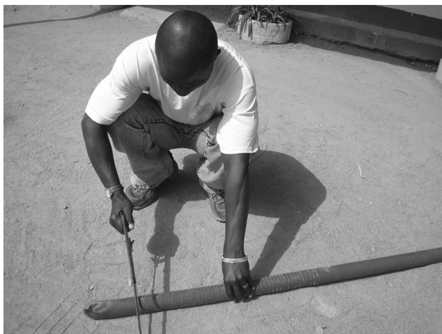
Preparation of rising main showing hand-cut slots and sealed end.
