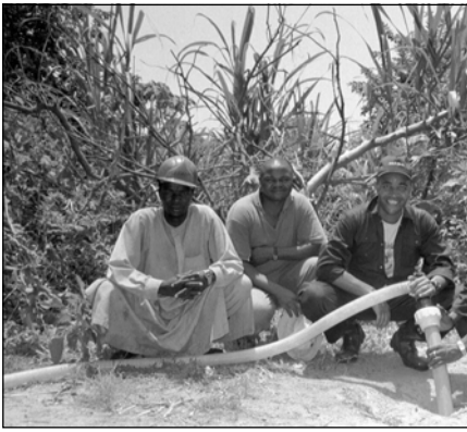
Rising main emerging from sediments, connected directly to pump suction.
