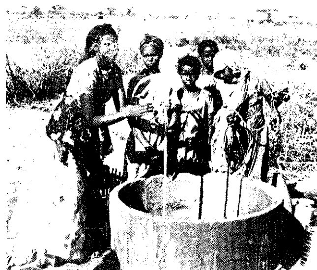
The rim of the well is brought above ground.
