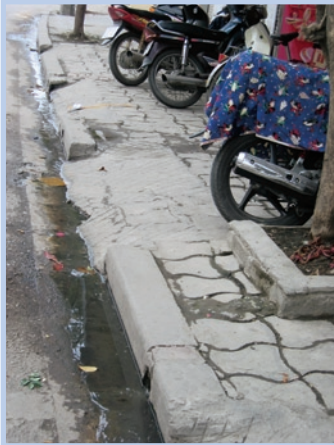
Photo2-1: Greywater discharge in Hanoi (photo: Sandec)
