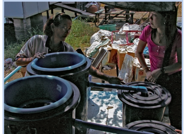
Photo 4-2: Mosquito nets used as coarse filter in a combined sedimentation/filtration system for greywater treatment in Bangkok's channel communities. The light blue basin can be removed and easily cleaned (photo: Sandec)
