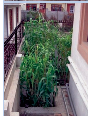
Photo 5-6: Vertical-flow planted filter shortly after completion (above) and in use (below) (photos: Shrestha R.R.)
