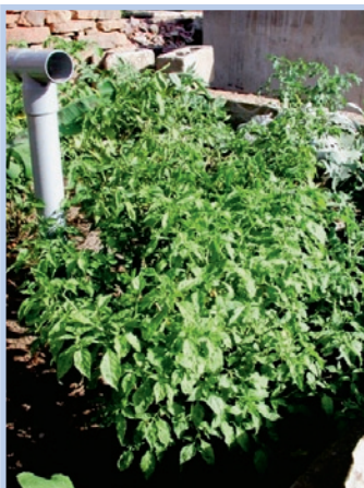
Photo 5-2: Planted greywater garden and aeration pipe (photo: GTZ)
