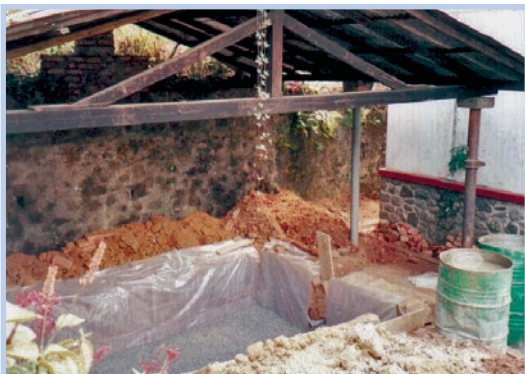
Photo 5-11: Construction of the percolation bed for subsystem 2 (photo: Harindra Corea E.J.)
