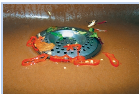
Photo 4-1: Kitchen sink screen to prevent solids from entering the treatment system (photo: Sandec)
