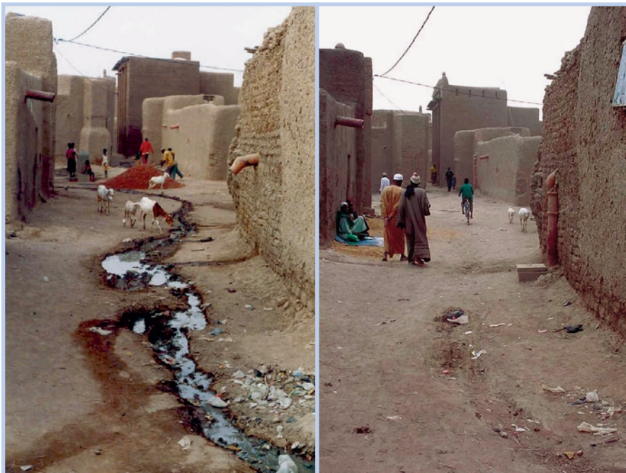
Photo 2-2: Djenné, Mali – The uncontrolled discharge of greywater has led to a deterioration of the streets, disease outbreaks, odour problems, and increased transport costs (left photo). The introduction of simple greywater infiltration systems as seen in the right photo on the wall, significantly improved the living conditions (photos: left, Alderlieste M.C., right, Langeveld J.G.)
