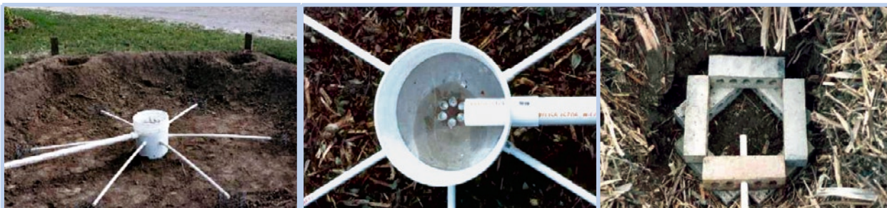
Photo 4-12: Greywater infiltration and irrigation system in Casa Juliana, Texas. Kitchen greywater is distributed via a hub to six small infiltration chambers irrigating papayas and bananas. The chambers are filled with mulch (photo: www.omick.net)
