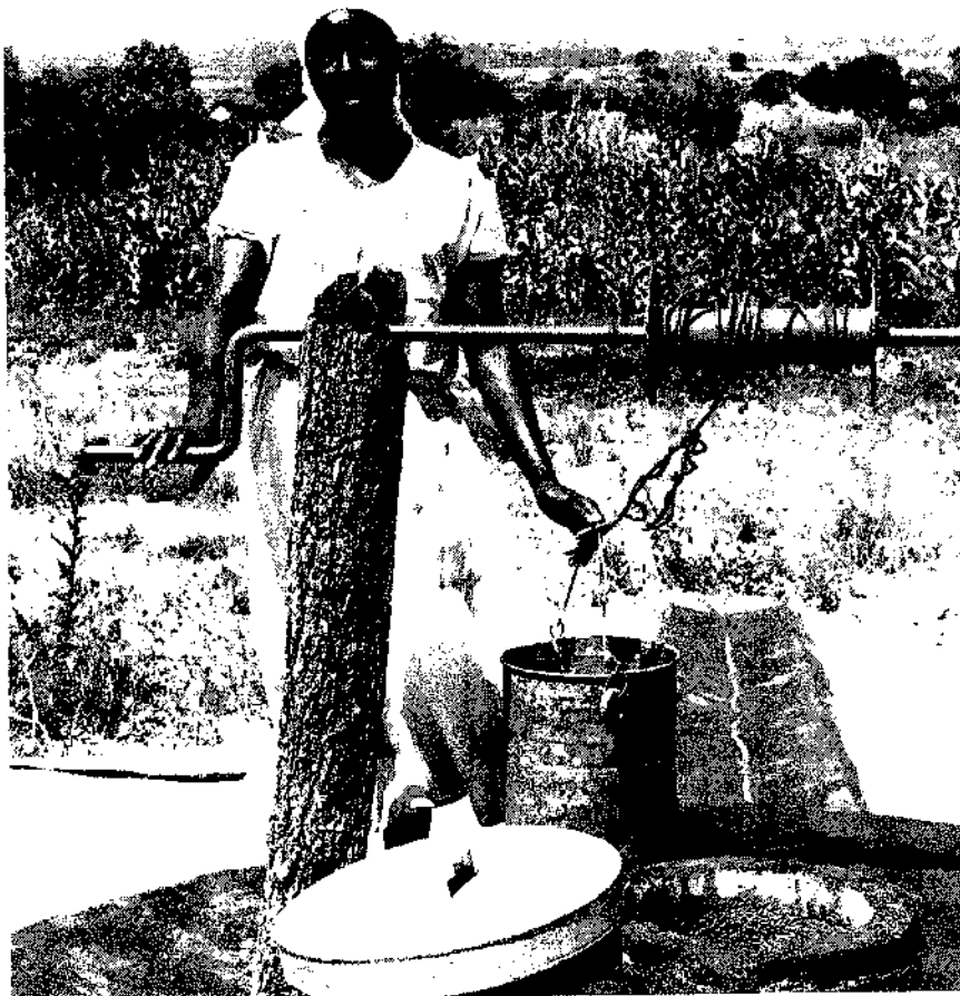
An upgraded family well showing the windlass mounted on stout poles, a raised collar forming part of the cover slab, and the tin lid provided in the 'subsidy'. Part of the apron and the water run-off can also be seen. The owners and users find this technology very acceptable.
