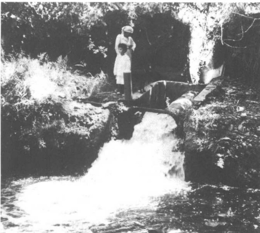
Figure 1. The turbine outlet, with the pipe built from oil drums.
