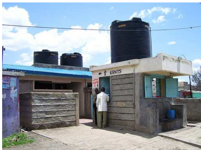
Figure 6: Naivasha public toilet with water kiosk. In front is the water kiosk that functions as an operator room. Customers pay at the side window of it, where the two people stand. Behind you can see the gents section of the toilet (source: C. Rieck, 2008) 4 .
