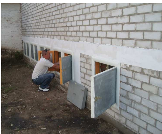
Figure 8: Inspection of the faecal chambers of a UUDT school toilet block in Nizhyn, Ukraine, constructed by the local NGO Mama86 (source: WECF, Claudia Wendland).
