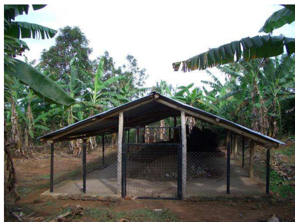
Figure 3: Drying shed for faecal matter from UDDTs at Kalungu School, Uganda. The caretaker has to take the containers with faeces from the UDDTs to this shed (source: EcoSan Club, 2009).
