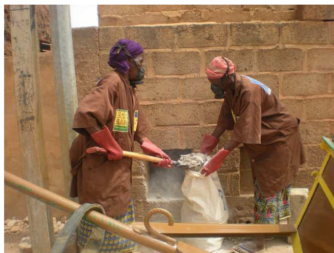
Figure 2: Two staff members from a service provider are emptying the faeces vaults of household UDDTs in Ouagadougou, Burkina Faso (source: Sandrine Tapsoba, 2009) 2 .
