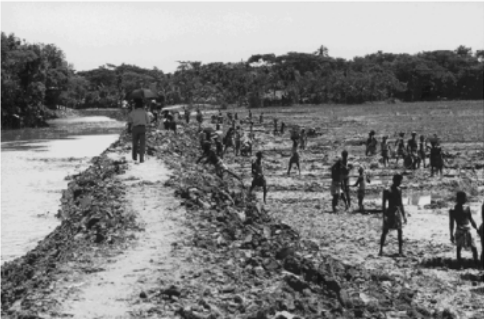
Construction of an emergency embankment in Bhola (Photo by D. Frans/Lineair)
