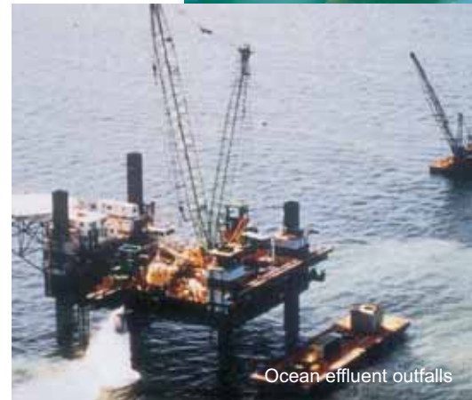
Seawater intakes and outfalls
