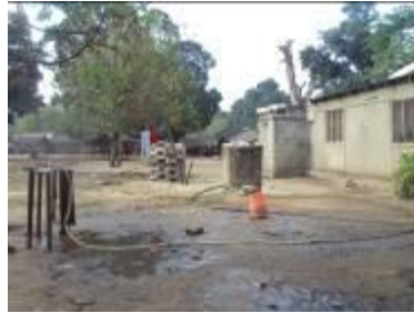
Photo 2: Water point in poor conditions
