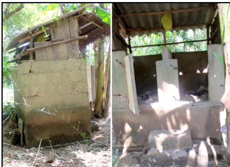
Figure 4.5 - Double-vault composting toilet in Trieu Do commune
