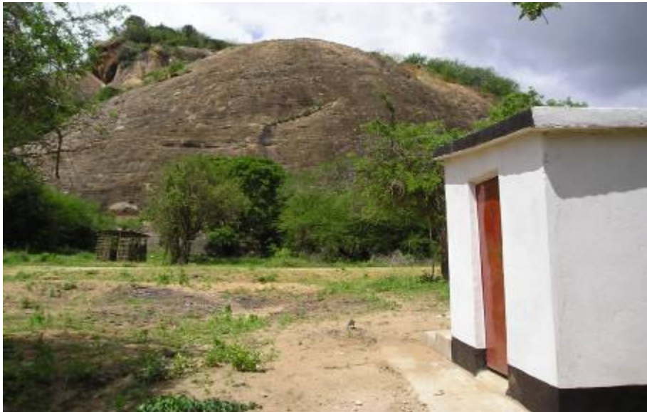
Rainwater harvested in Yawia Rock Catchment Dam is gravitated down to a kiosk.
