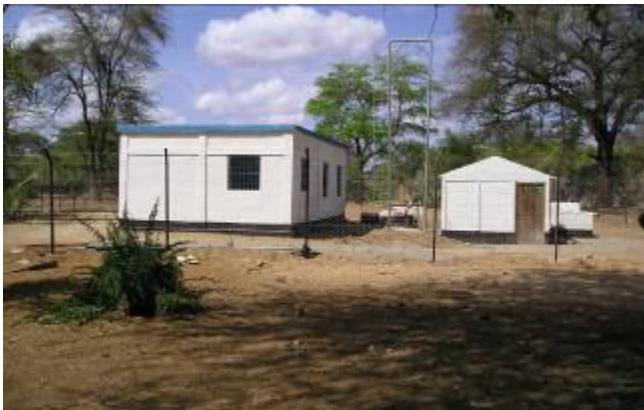
Kalambani pump house at Thua riverbed.
