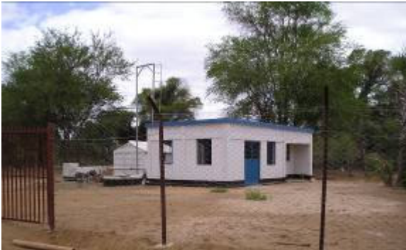
Kalambani pump house at Thua riverbed.
