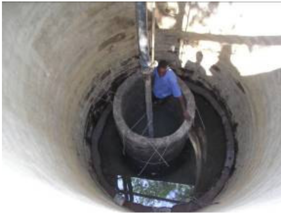
The river-intakes at Kisasi, Mbitini and Ikoo consists of a small diameter hand-dug well sunk inside a wide-diameter hand-dug well.
