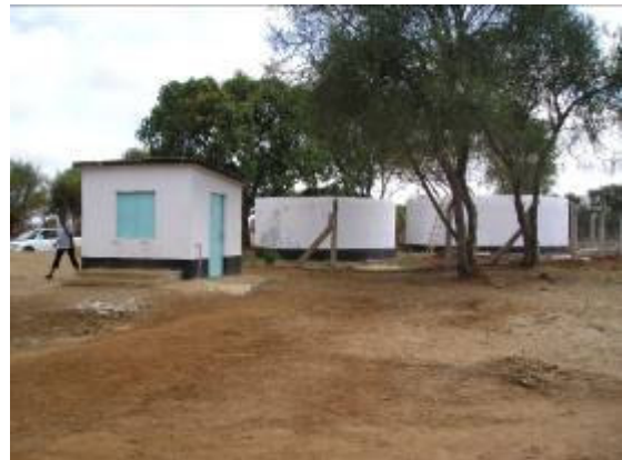
Water kiosk and water tanks at Kisasi
