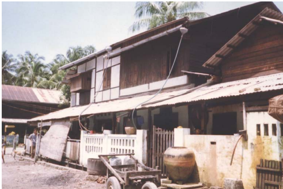
Hosepipes attached to funnels drain water from gutters to a series of jars.
