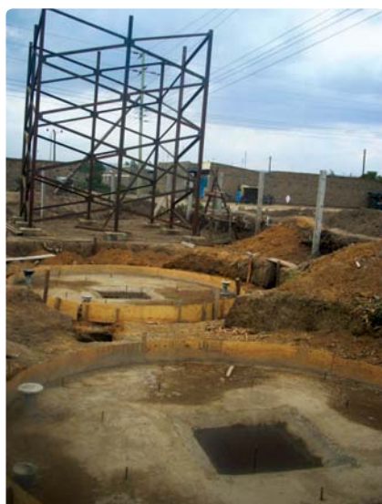
Water tank construction, Karagita
