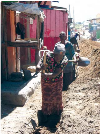
Digging a pipeline trench in Kamere
