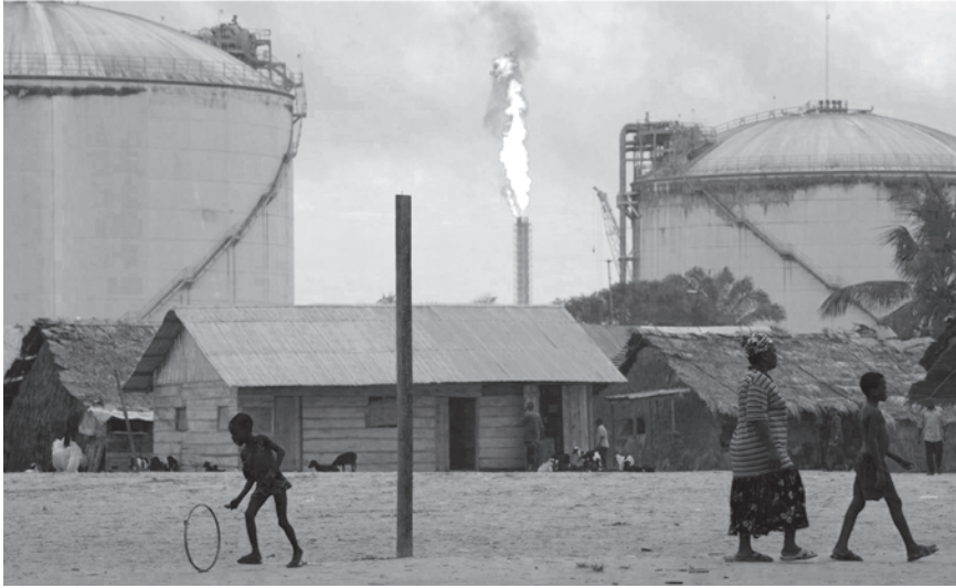
IMAGE A1 ExxonMobil gas plant in the village of Finima, Nigeria
