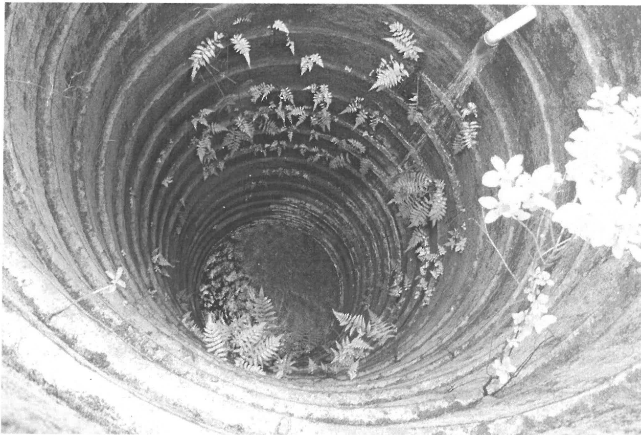
Konkodi Bhat's well showing inlet pipe on the right.
