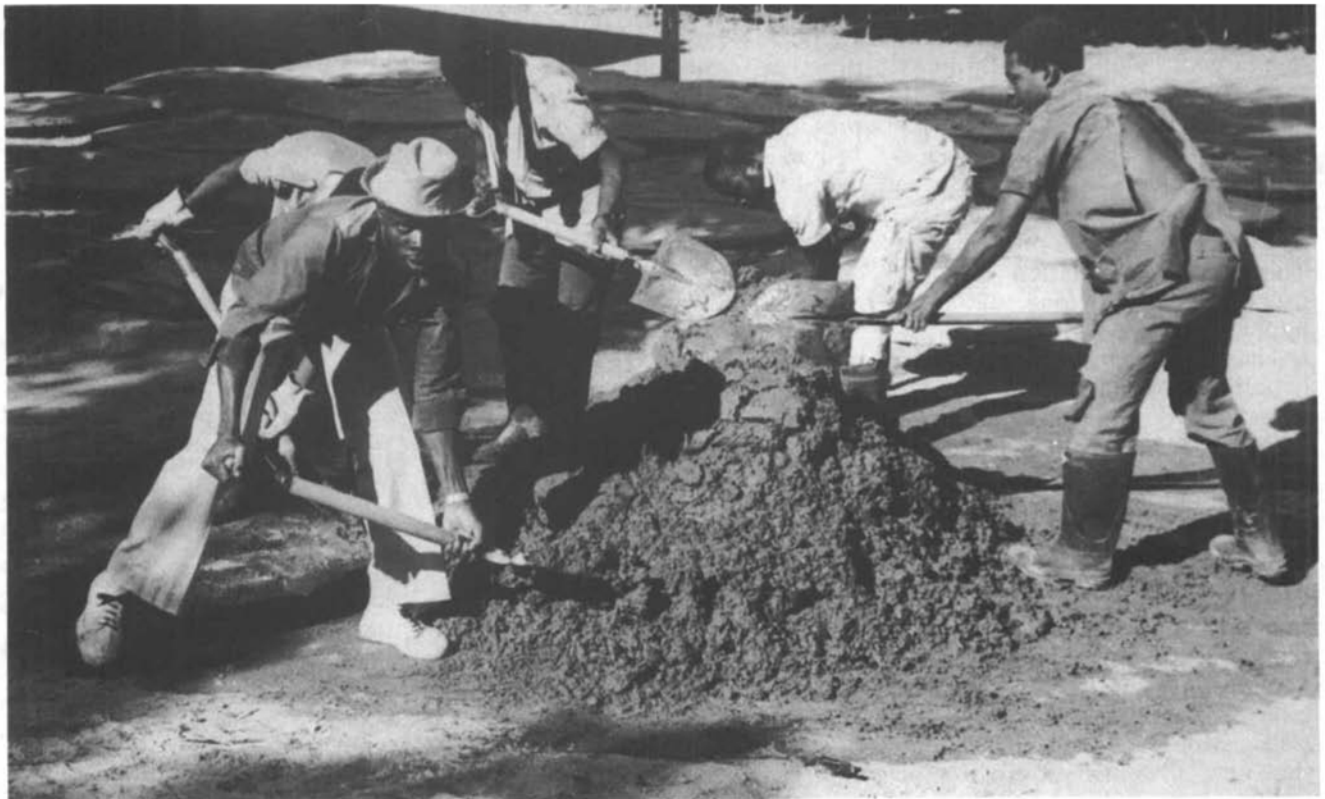
Mixing cement with which to build slabs at Maxaquene workshop.
