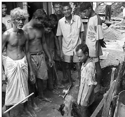
The water connection and meter is fitted.
