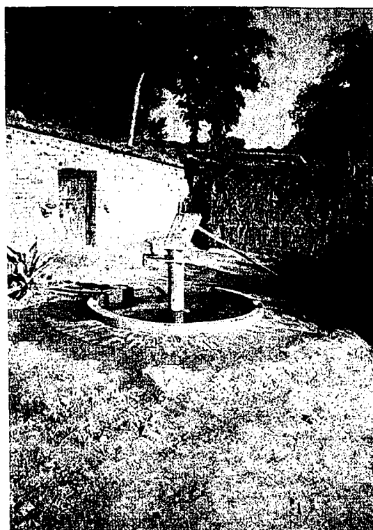
India Mark II handpump in Materiya hamlet of Paigapur village, Gonda District
