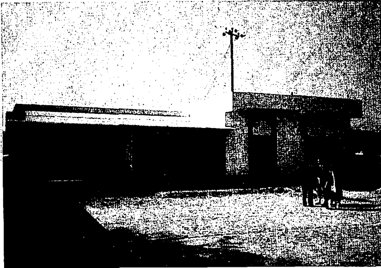
Jal Nigam godown in Atrauli Block, Aligarh District, constructed under the IDC programme
