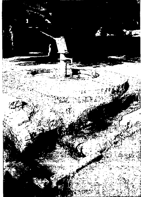
Handpump with brick-on-edge pavement and drainage facilities with soak pit at roadside. Jakhera village, Atrauli Block, Aligarh District.
