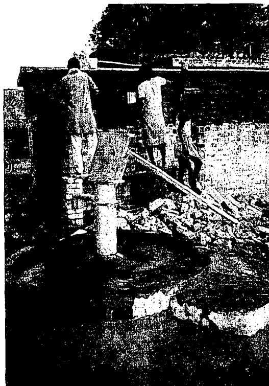
View of sanitary school latrine in Bachhaon village under renovation; India Mark II handpump in foreground
