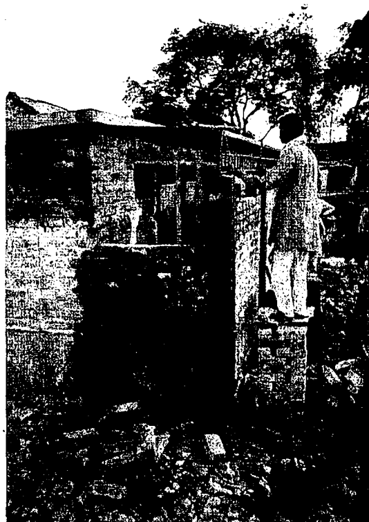
Renovation of school sanitary latrine going on; Bachhaon village, Varanasi District
