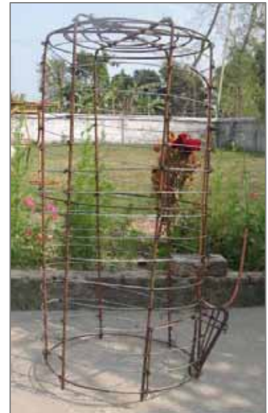
Figure 3: Reinforcement of ABF
