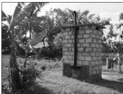
A compost toilet built in Hambanthota, 2006
