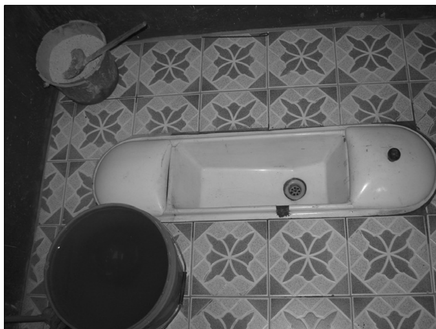
The compost toilet (eco solution, India model) showing on one side the water bucket and on the other an ash bucket
