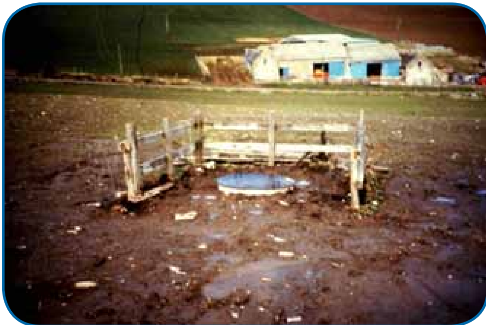
Borehole with no protection from livestock, Scotland
