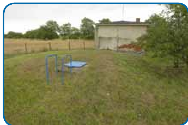
Properly maintained well head, source supplying small village in Southern Moravia, Czech Republic © National Institute of Public Health, Prague (Czech Republic)/ Frantisek Kozisek
