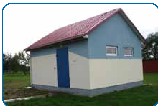
Well house of a rural, public water supply, Lithuania © UBA, Dessau-Roßlau (Germany)/ Oliver Schmoll
