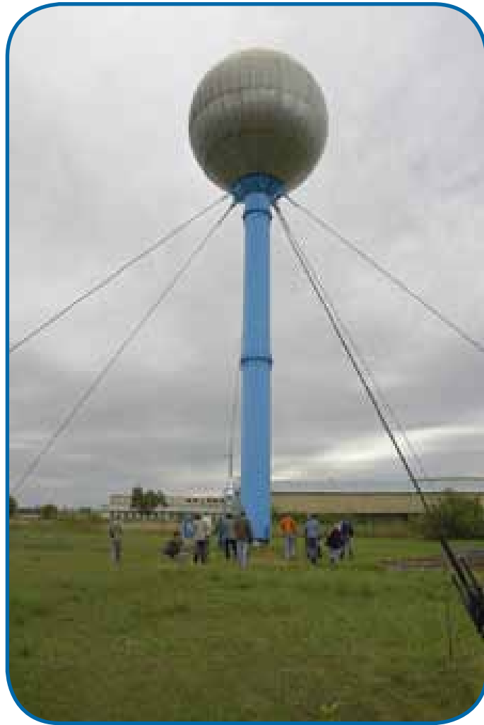
Water reservoir tower supplying small village in Southern Moravia, Czech Republic
