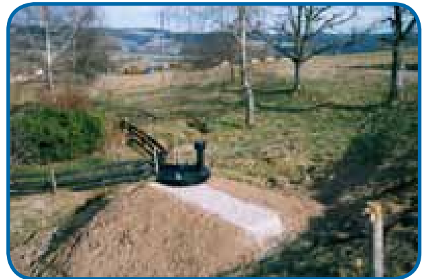
Well after refurbishment
