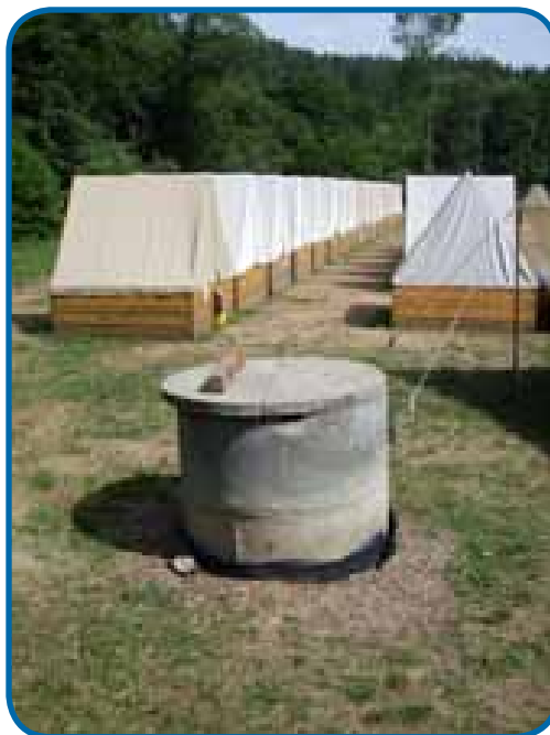
Well supplying summer youth camp, with improperly sealed cover, Western Bohemia, Czech Republic
