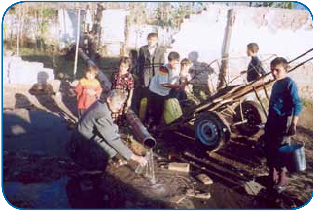
Damaged water supply system in Farhor district, Khatlon region, Tajikistan
