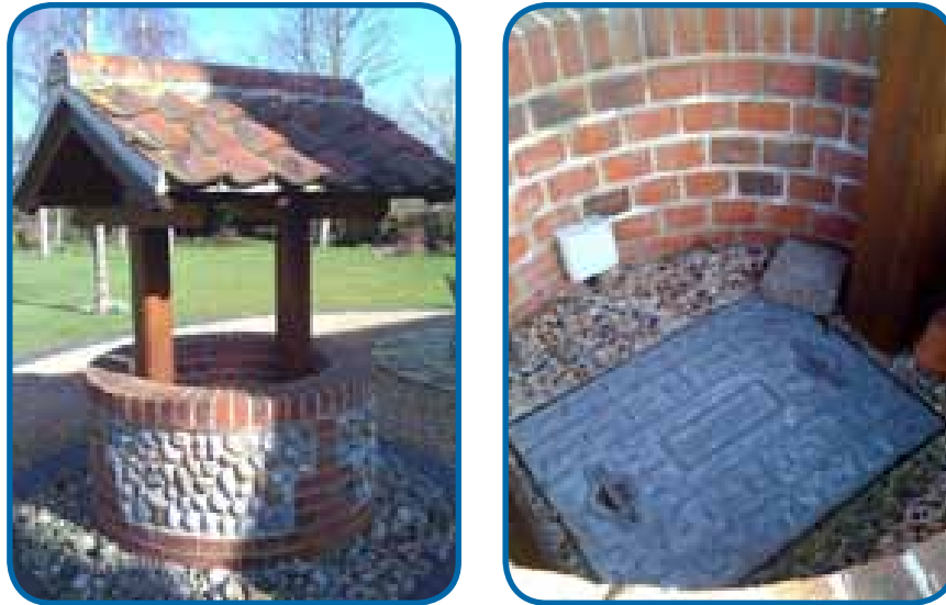
Steel inspection cover for a modern household well, Norfolk, England © University of East Anglia, Norwich (United Kingdom)/ Helen Risebro
