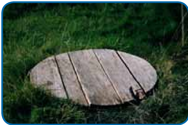
Wooden cover of well before refurbishment
