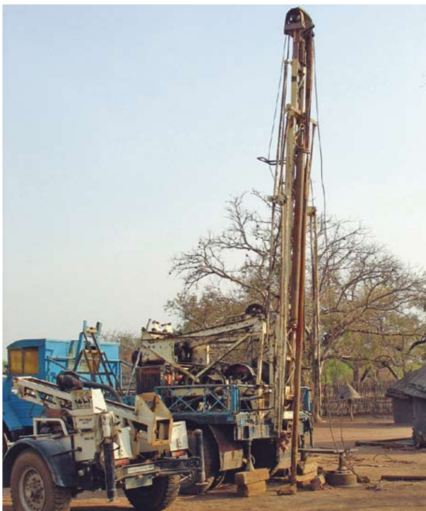
DTH hammer rig in Sudan
