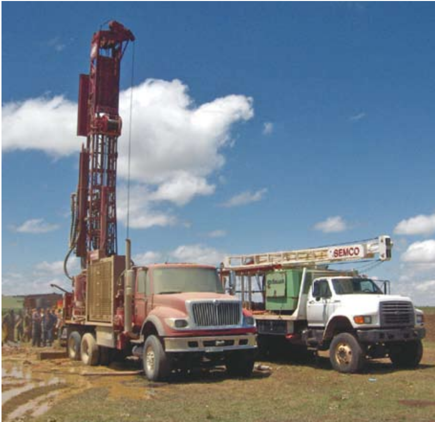
TWWD Ingersoll drilling rig
