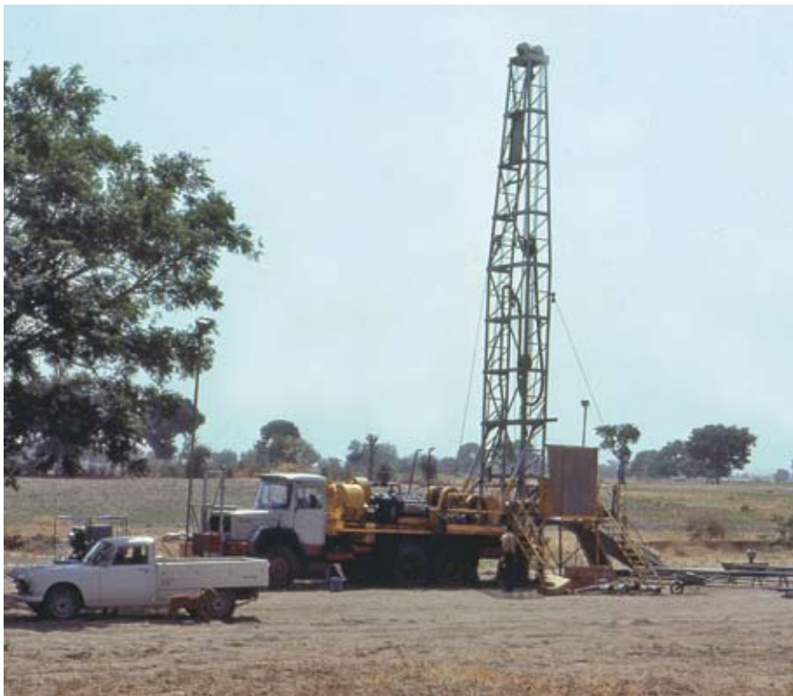
Deep drilling in Nigeria
