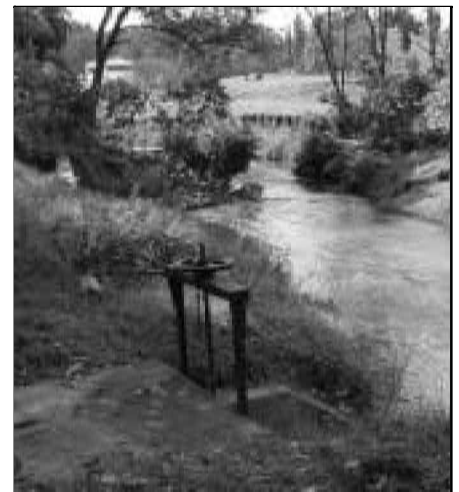
The outlet of treated water into La Mosca creek
