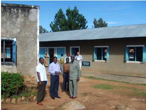
LGDCG funds are used to construct new classrooms
