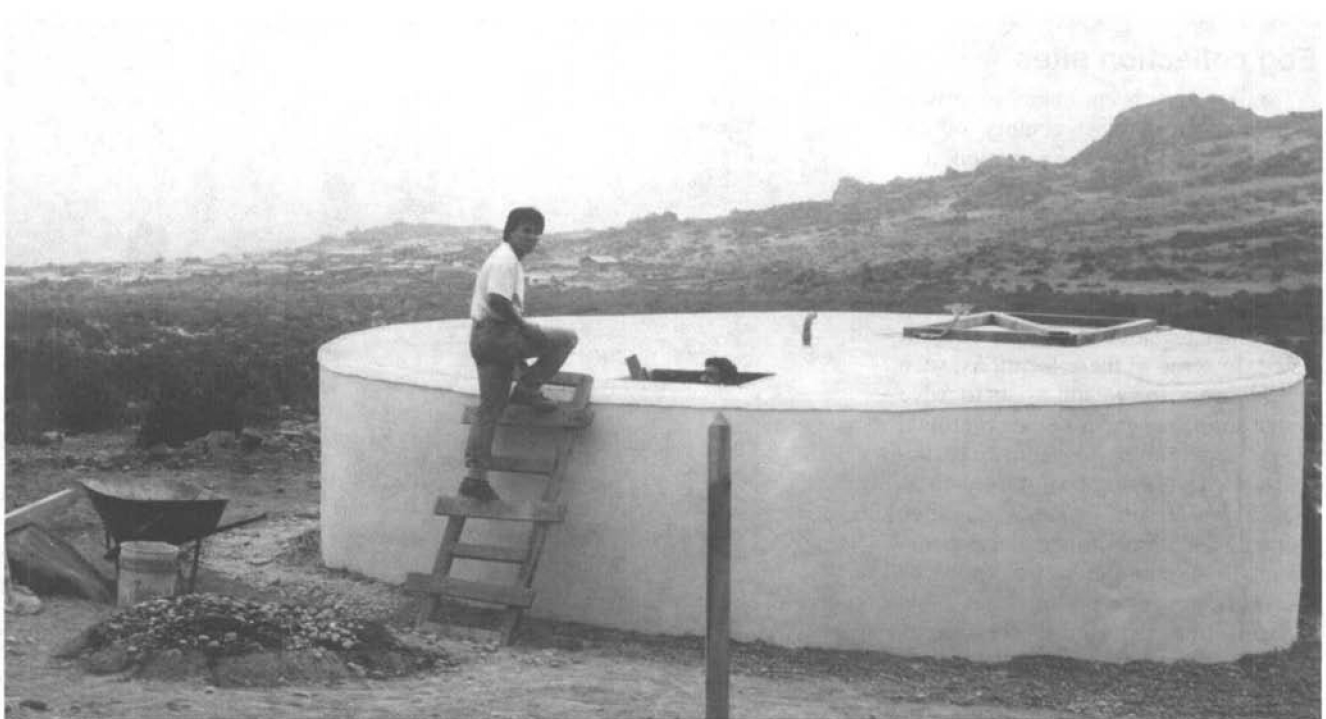
The 100 000-litre fog water storage tank near the village of Chungungo on the northern coast of Chile.
