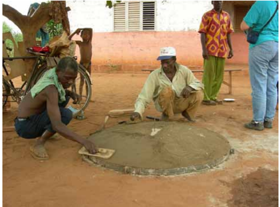
Trained mason building casting slab on-site for new customer.
