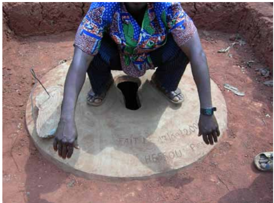
A newly-constructed slab.
