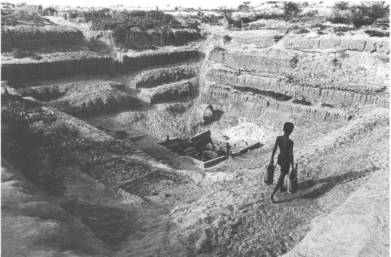
Traditional methods of water supply and irrigation exist all over the world. This hand-dug inverted 'cone' in Mali was built during a recent drought.
