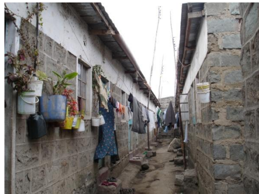
Figure 4: Typical concrete & brick dwelling
