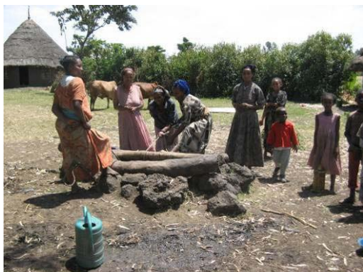
Figure 3-8 Timber parapet and dry-stone topping, Meskan
