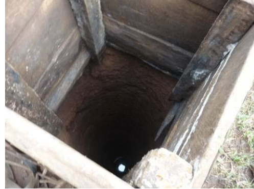
Figure 3-2 Timber well headworks A. Wendo
