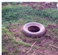
Figure 3-11 Spare tyre parapet installed where a broken rope pump has been removed, Chench
