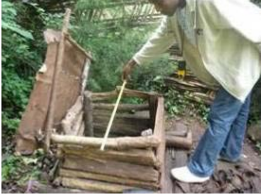
Figure 0-2 Aleta Wendo - wooden well-head protection - measuring the well diameter
