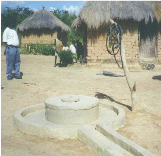
Figure 6-2 Example of parapet, apron with lip and drainage channel using 2 bags of cement. A minimum protection level?
