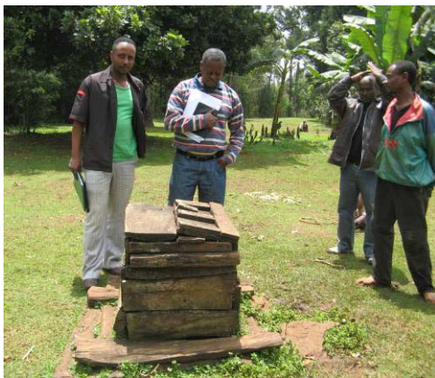
Figure 3-3 Timber well parapet in Aleta Wendo
