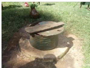
Figure 3-5 Oil drum and apron, Boloso Sore
