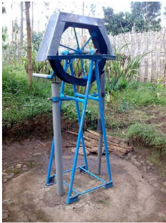
Figure 5-2 Good rope pump, but installed below ground level, with no drainage or spout, so high opportunity for spilled water to seep back into the well
