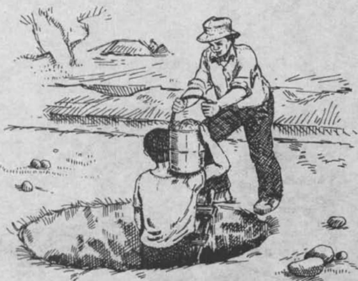
Figure 4: Digging an infiltration well
