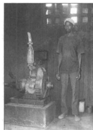
The mechanic and the 1hp pump motor for the borehole at Diass.
