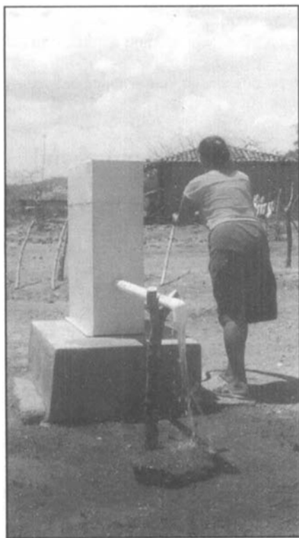
A woman uses a 'rope and washer' pump that has been modified and improved by AHJASA.
