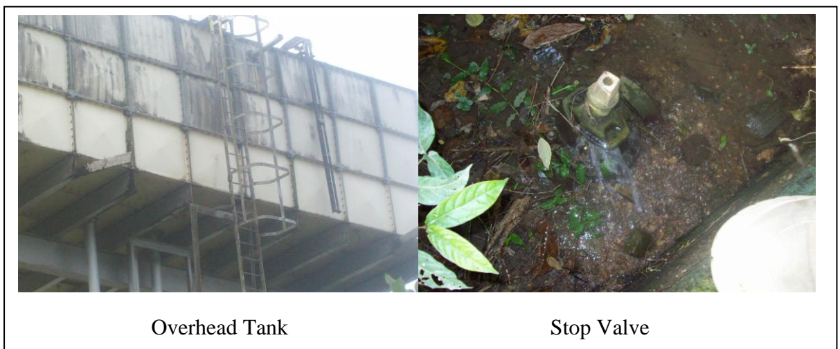
Figure 3.1: Pictures Showing Leakages
