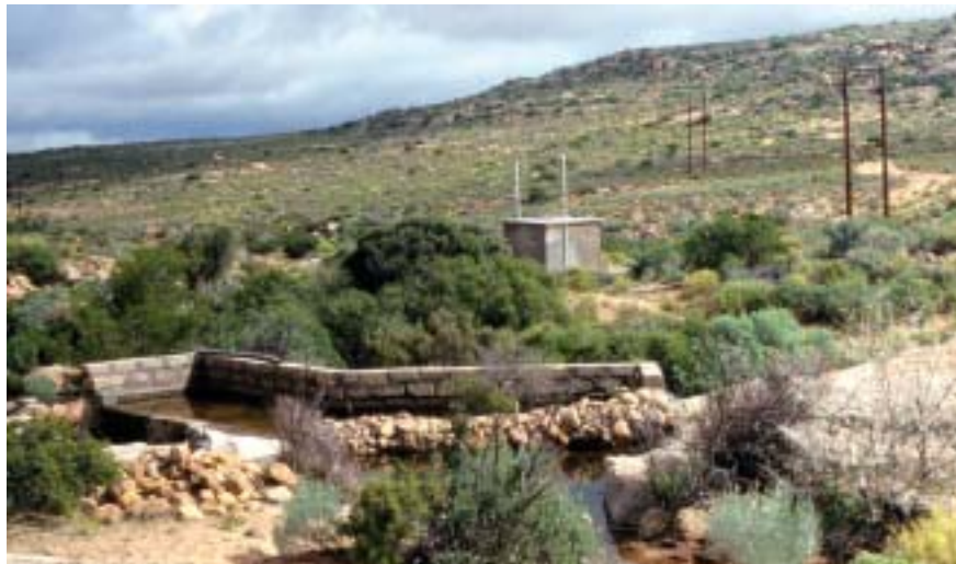
Figure 2. Filter for ephemeral spring, with injection borehole in background, Karkams (Murray & Tredoux, 2002c).
