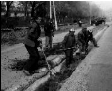
Cleaning drainage system Osh, Kyrgyzstan
