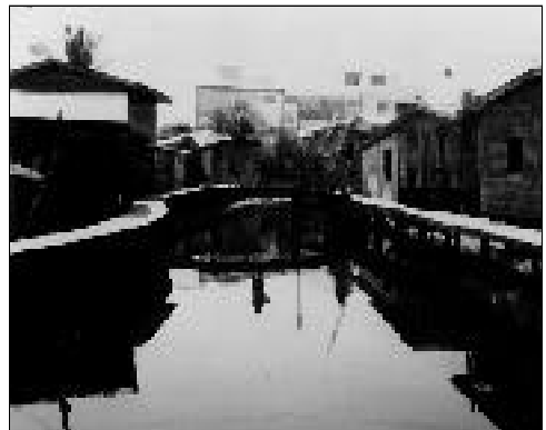
Local slum communities cleaned and dredged this canal and built a community boardwalk in Thailand
