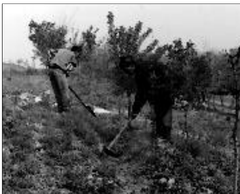
Clearing the ground for a new irrigation system and recently planted trees, Osh, Kyrgyzstan
