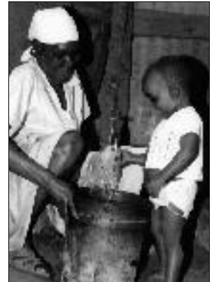
S-Corner water supply project, St. Joseph Road, Jamaica
