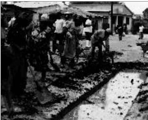
Women clearing new community drainage system, Hanna Nassif, Dar es Salaam, Tanzania
