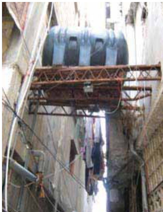
An elevated private water tank to cope with the high built-up density in Tawari
