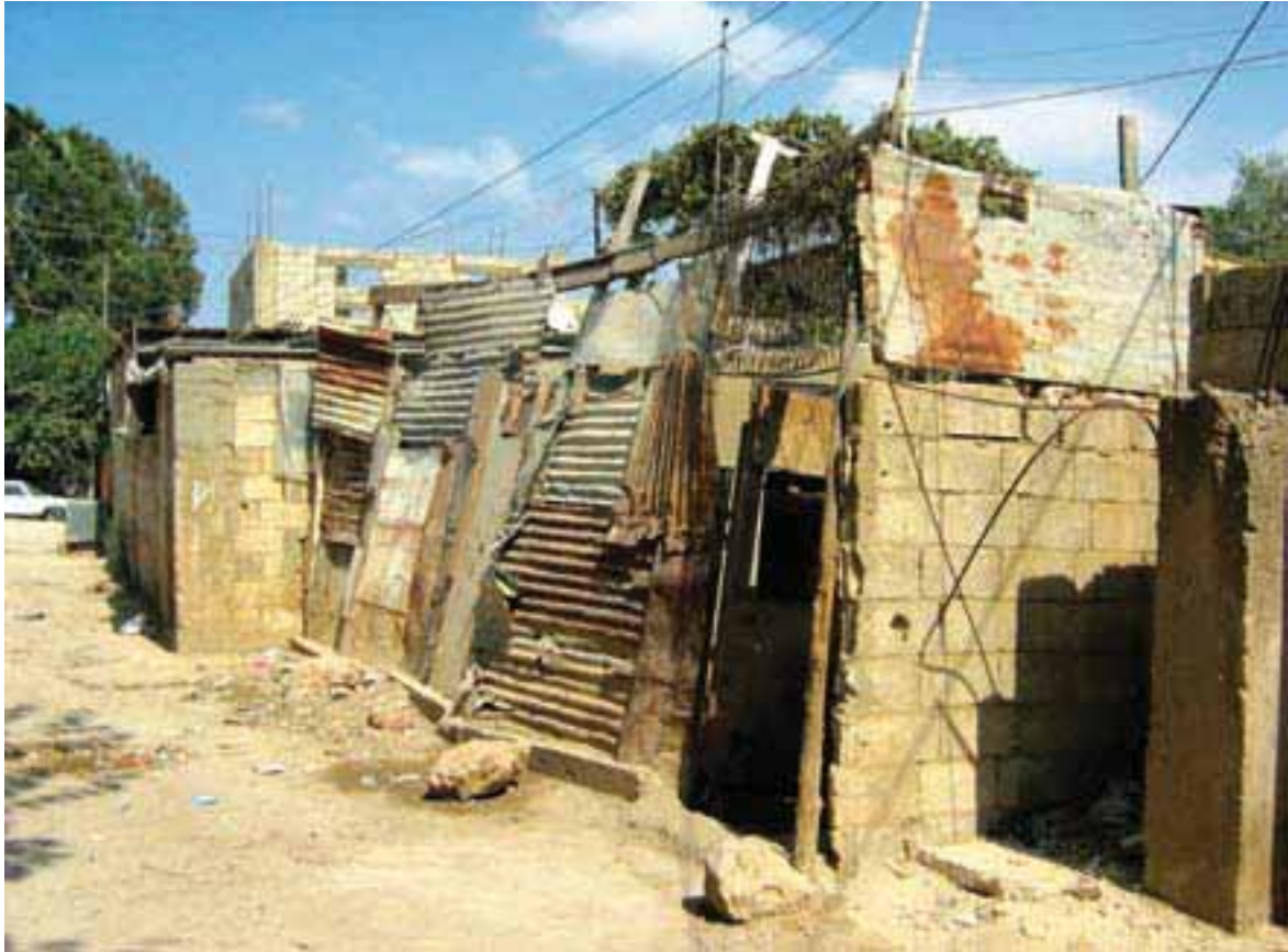
Living conditions are generally deteriorated in the AAs (Tallet el Mankoubin AA around Beddawi Camp in North Lebanon)
