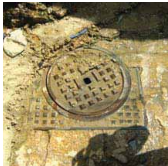
Manholes installed by UNICEF in Mouhajarin
