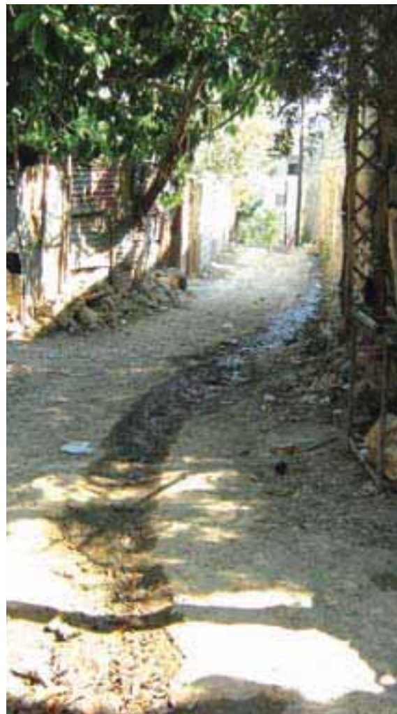
Sewage floods on the streets due to the lack of a sewage network in Tallet el Mankoubin
