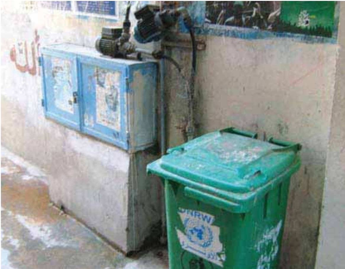
UNRWA informally extends some BUS to the AAs, note the collective water manifold and the solid waste container in the AA of Mieh Mieh Camp
