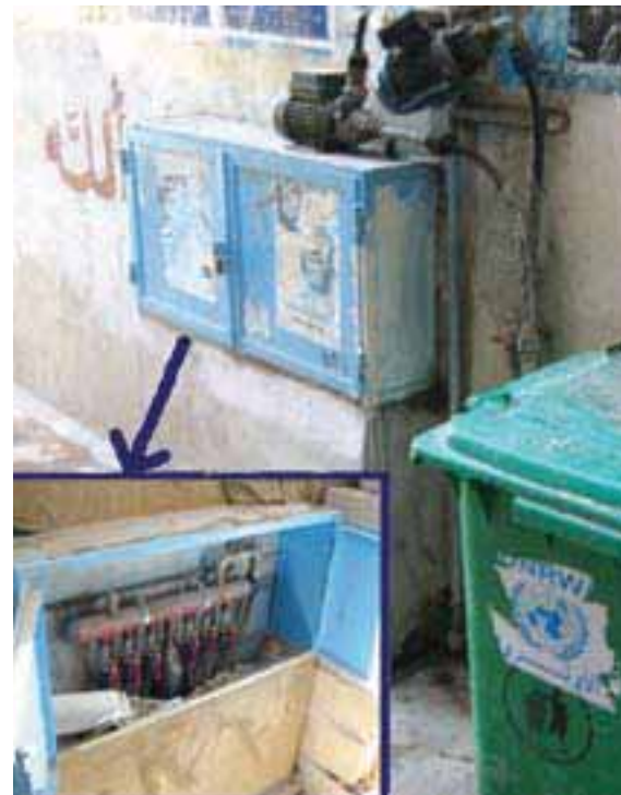
Collective water manifold installed by UNRWA as part of a WATSAN project extended to Mieh Mieh AA
