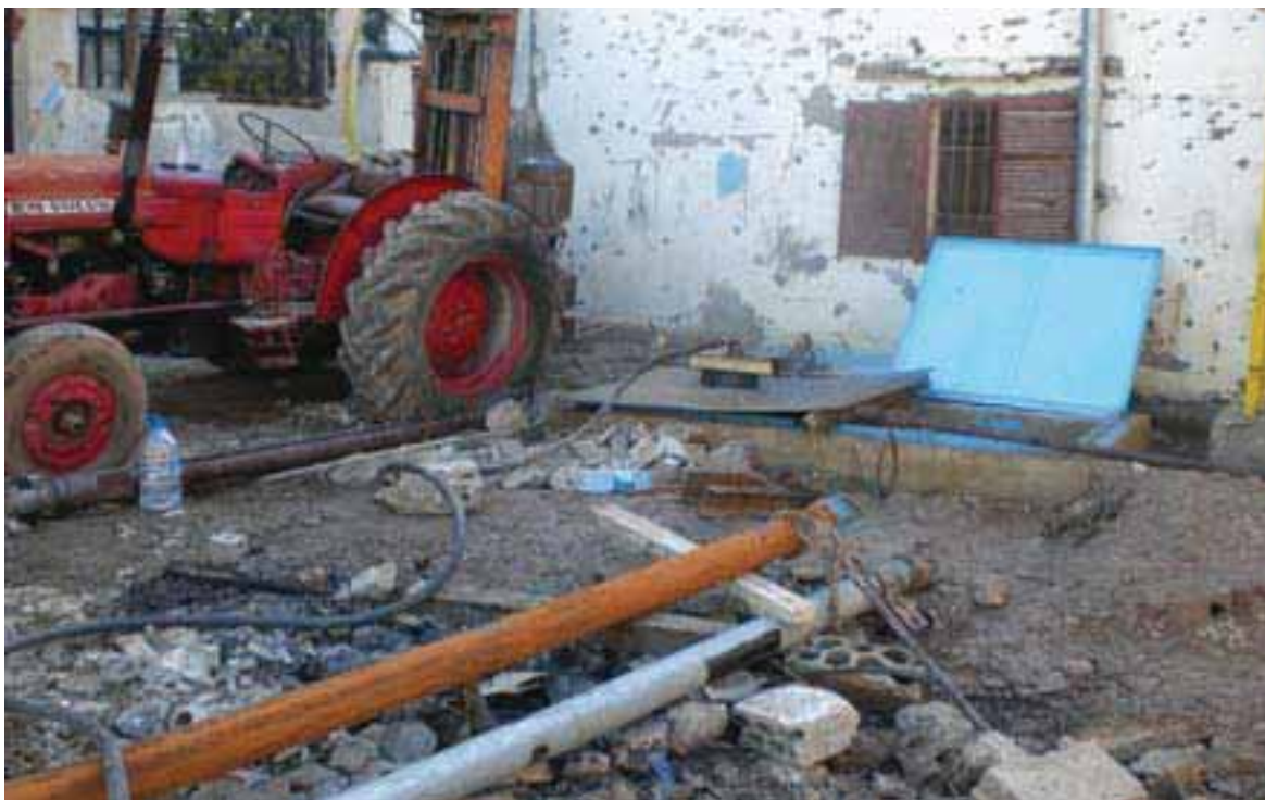
Drilling of water wells in NBC AA (Source NBRC)
