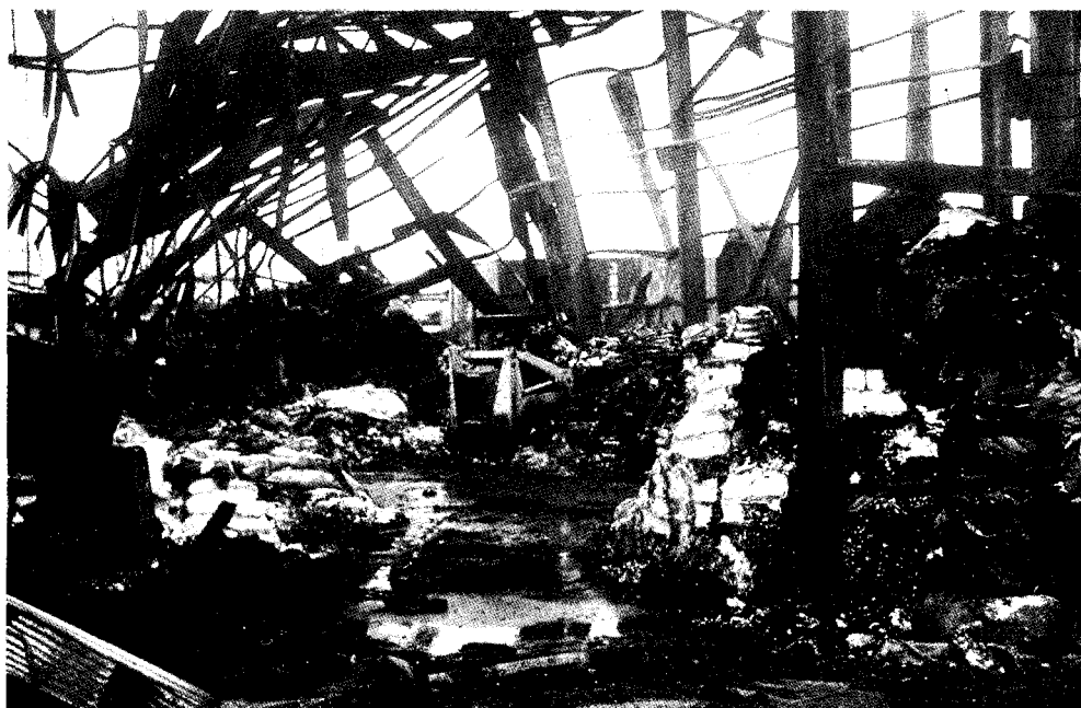
Consequences of fire in a factory, Melbourne, 1985. Photo : F. BALKAU
