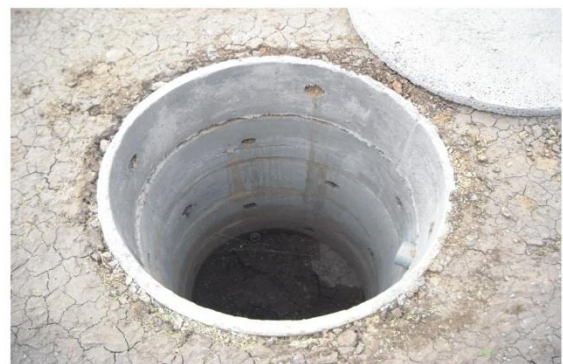
Cement rings pit lining
