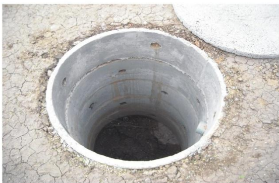
Cement rings pit lining
