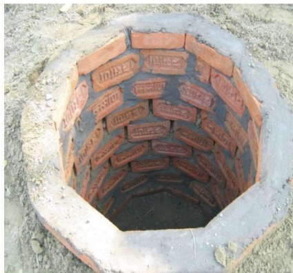
Pit Lining (Bricks)
