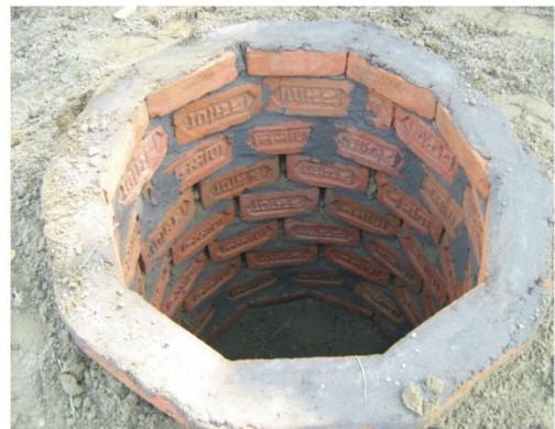
Pit Lining (Bricks)
