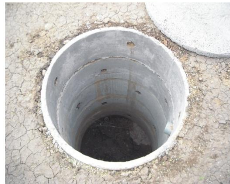
Cement rings pit lining
