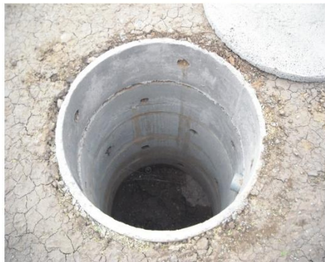
Cement rings pit lining
