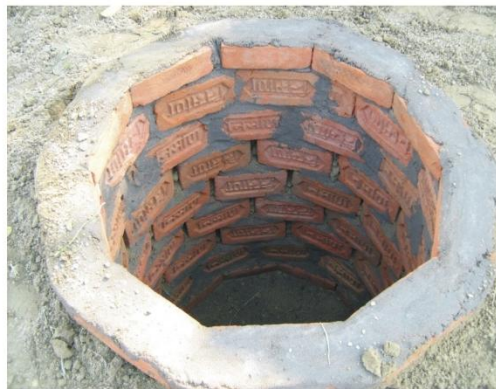
Pit Lining (Bricks)
