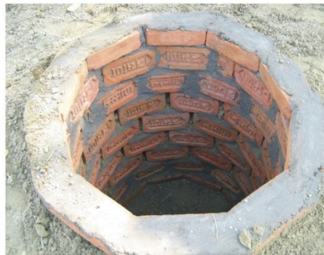
Pit Lining (Bricks)
