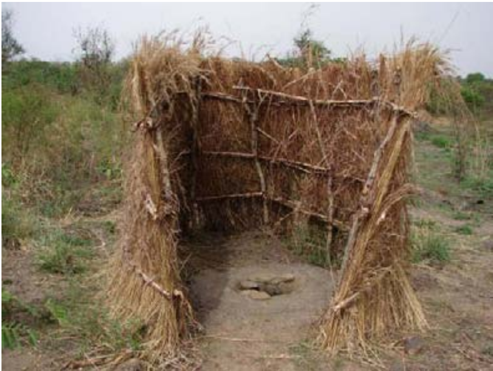
Simple Pit Latrine in Arua
