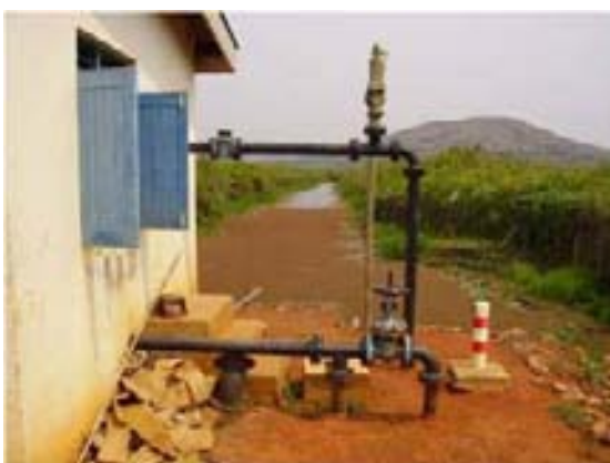
Figure 11.1 Intake at Lyantonde Water Works - Covered by Algae
