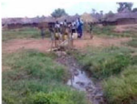
Poor Drainage at Water Point in Kitgum
