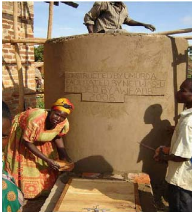
A woman constructing a rainwater harvesting tank in Bugiri District
