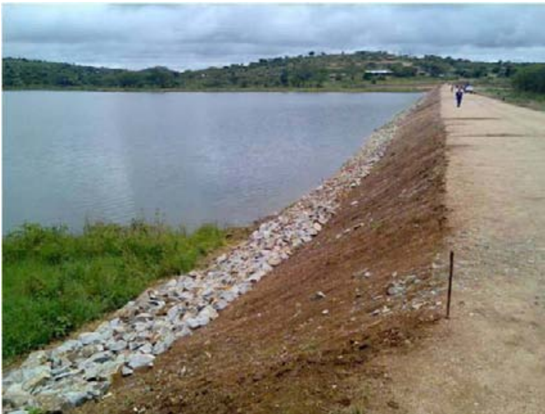
Reconstruction of Kakinga Dam in Sembabule District in progress, March 2008
