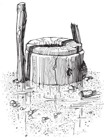
Figure 15.3. A damaged well, showing cracks in the walls
