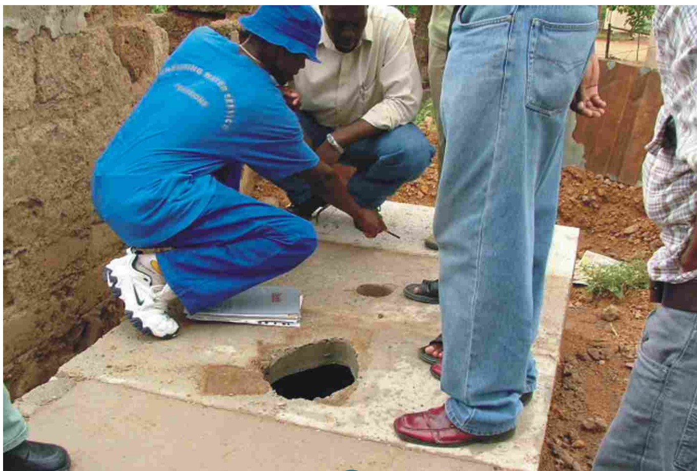
Builders laying the slab
