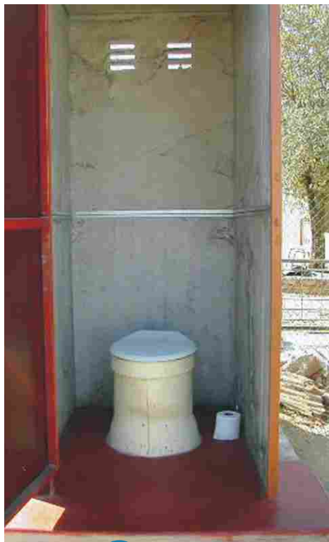
Inside view of a new VIP toilet
