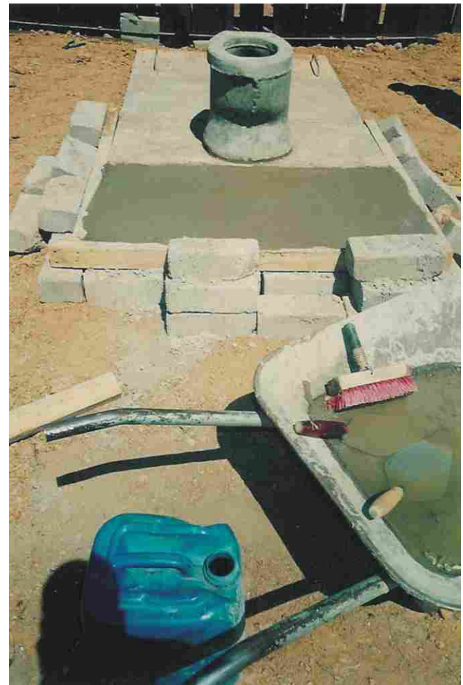
Building of the VIP toilet in progress
