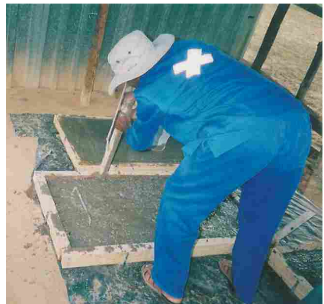
Slab casting process
