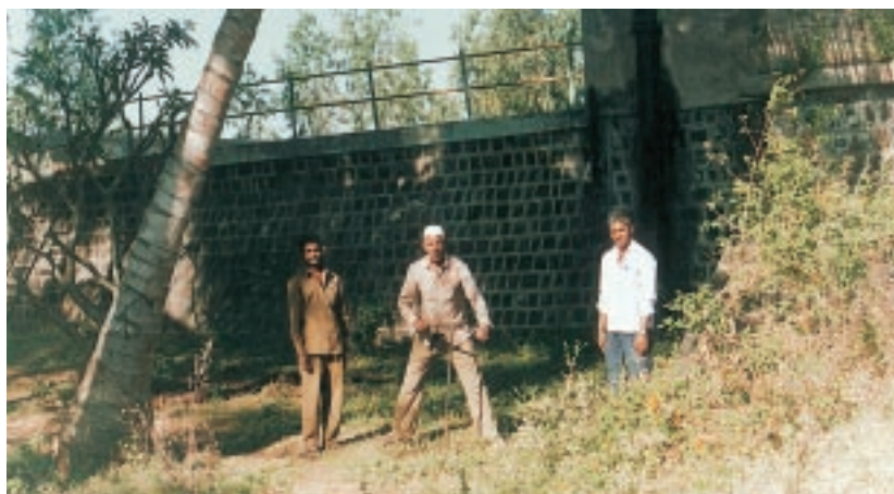
A caretaker opening the reservoir valve to release water
