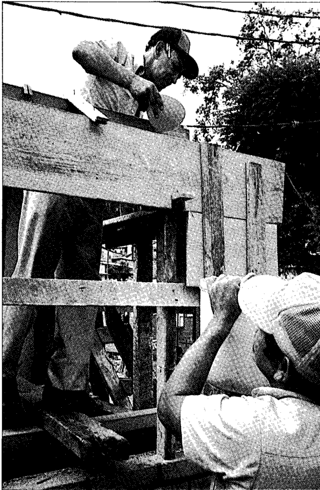
Courtesy of Cooperative Housing Foundation
