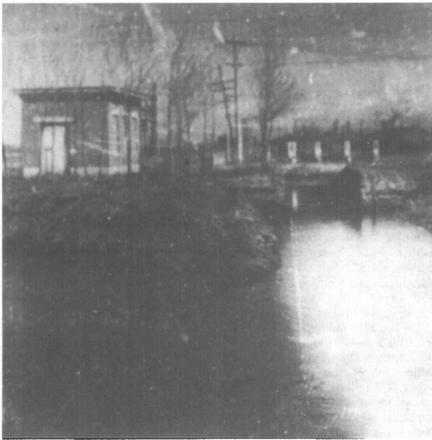
Waste water is diluted in a plant like this one in a suburb of Fushun City, and is then used for irrigation.
