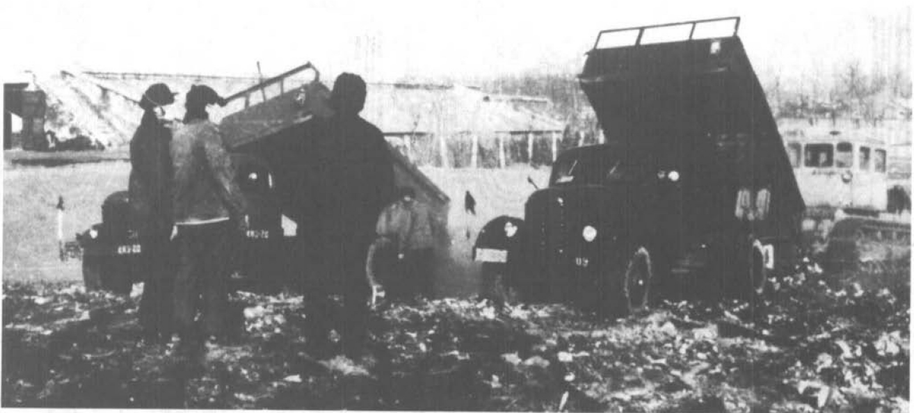
The disposal of domestic rubbish must be monitored to ensure that groundwater is not polluted as a result.
