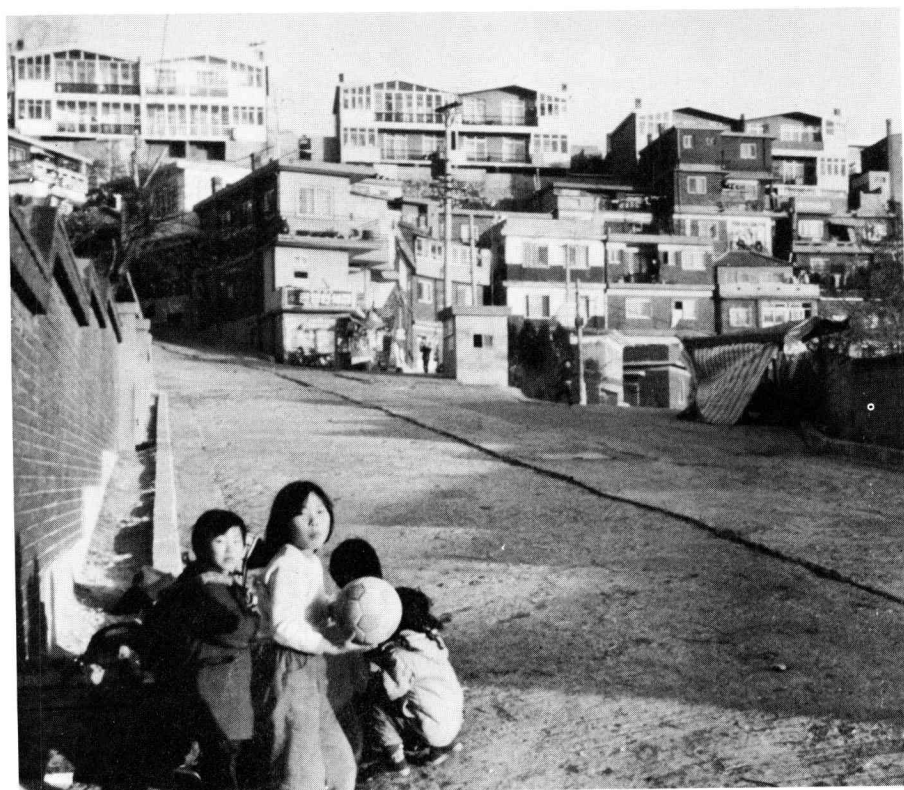
Fig. 11. Self-help access lane in Chulsae community (12 m wide and 350 m long).
