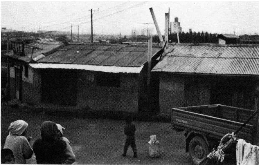
Fig. 3. Partially improved houses in Madong community.
