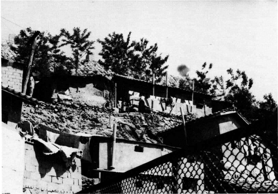
Fig. 14. Houses in Chulsae before improvement.
